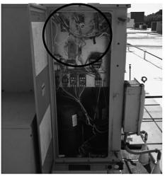
Model PACE2 retrofits with optional return-air sensor kit, installed in package unit control panel. Photo courtesy of PaceControls LLC.
